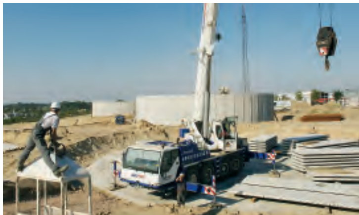
Construction of one of the 40 fermenters in Penkun
