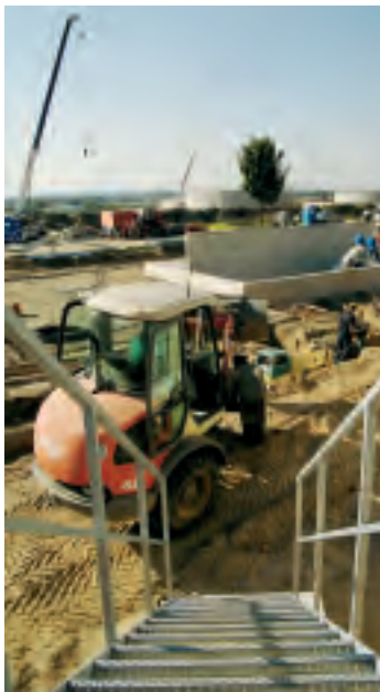
2A total of 25,000 cubic metres of concrete are being processed.
