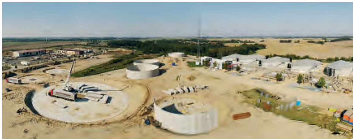
40 standardised 500kw modules make 20 mw – that is the largest biogas- plant- park of the world.
